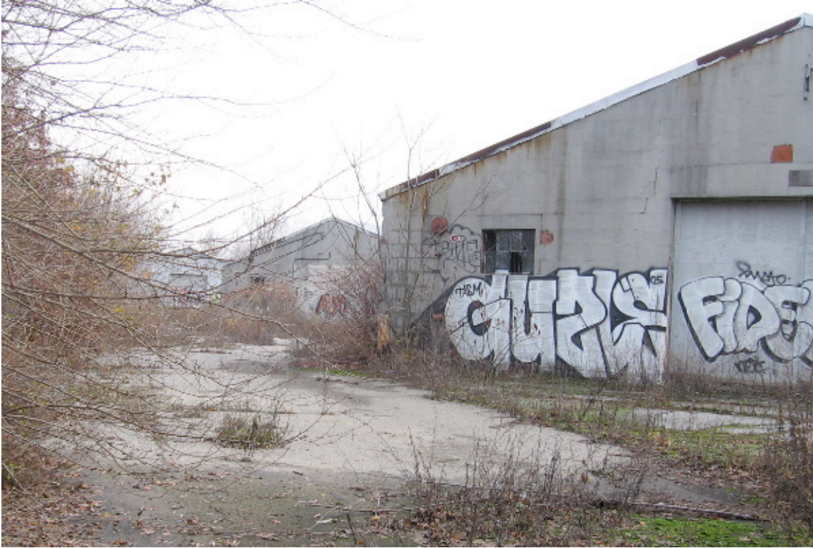
Buildings on the GSA parcel
