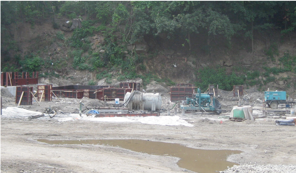
Construction at Former Marble Quarry Landfill brownfield, Tuckahoe, New York 1
