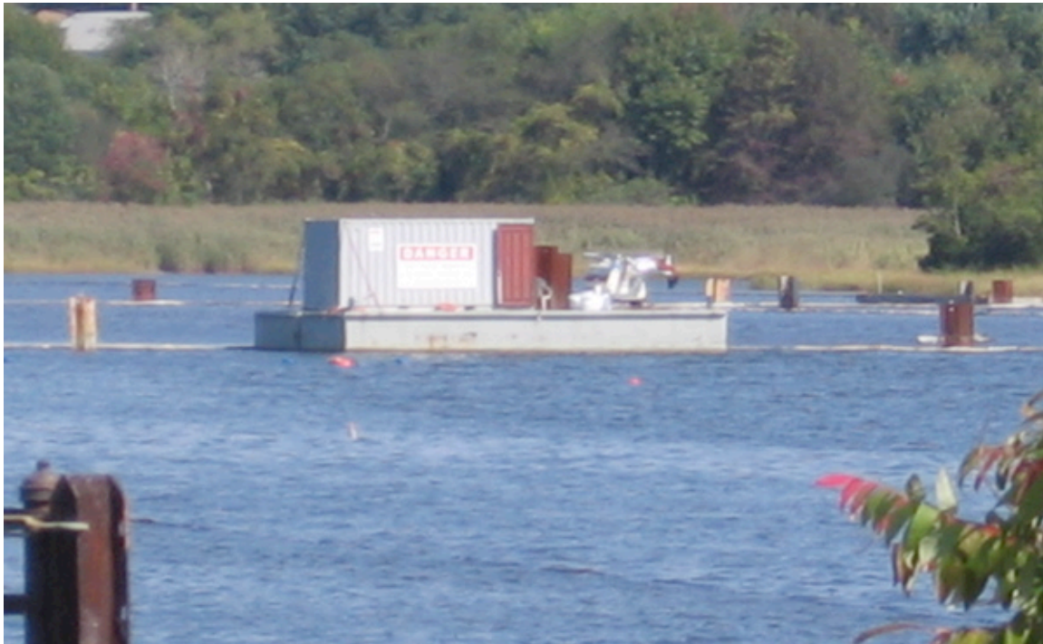
In New Bedford Harbor, Massachusetts the dredge is towed by cables from the shore
