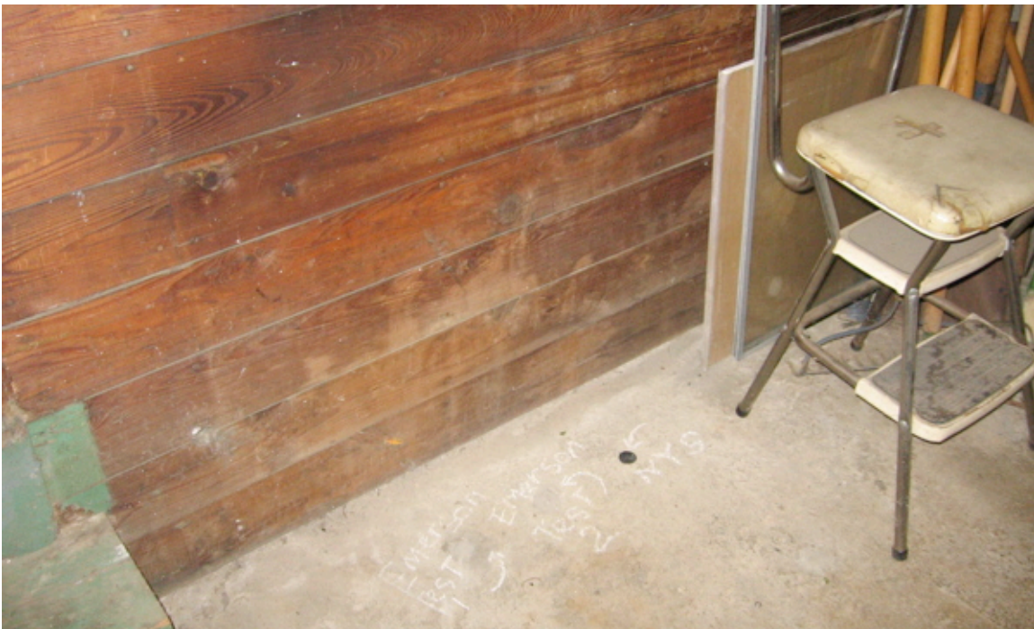
Sampling hole in an Ithaca, NY basement slab
