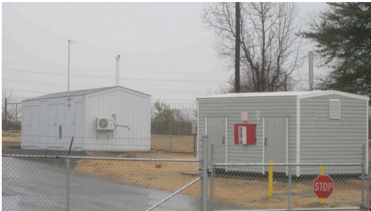
Treatment Systems on Kaba-Ilco Property
