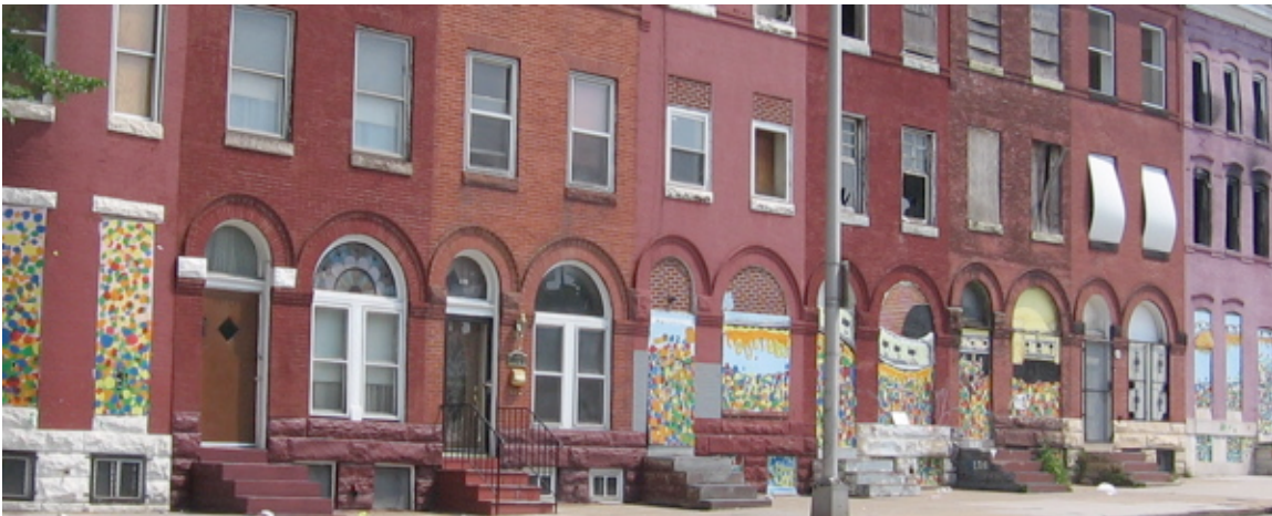
Occupied homes and bricked-up units with artwork
