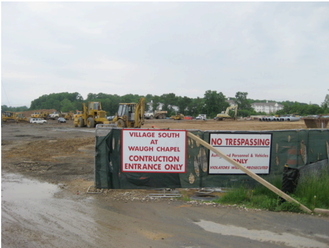
Turner Pit Construction Site—May, 2011
