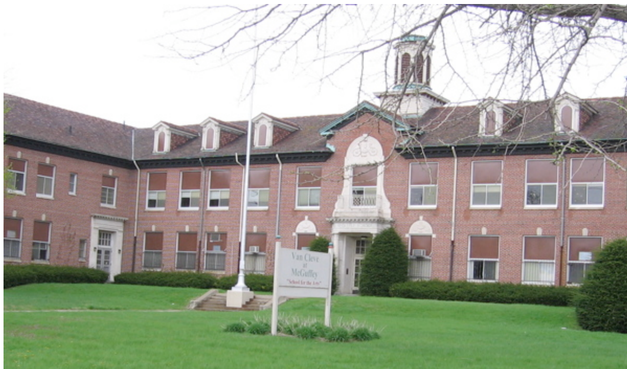
Van Cleve at McGuffey School in Dayton Ohio, Closed in Part Due to Vapor Intrusion
