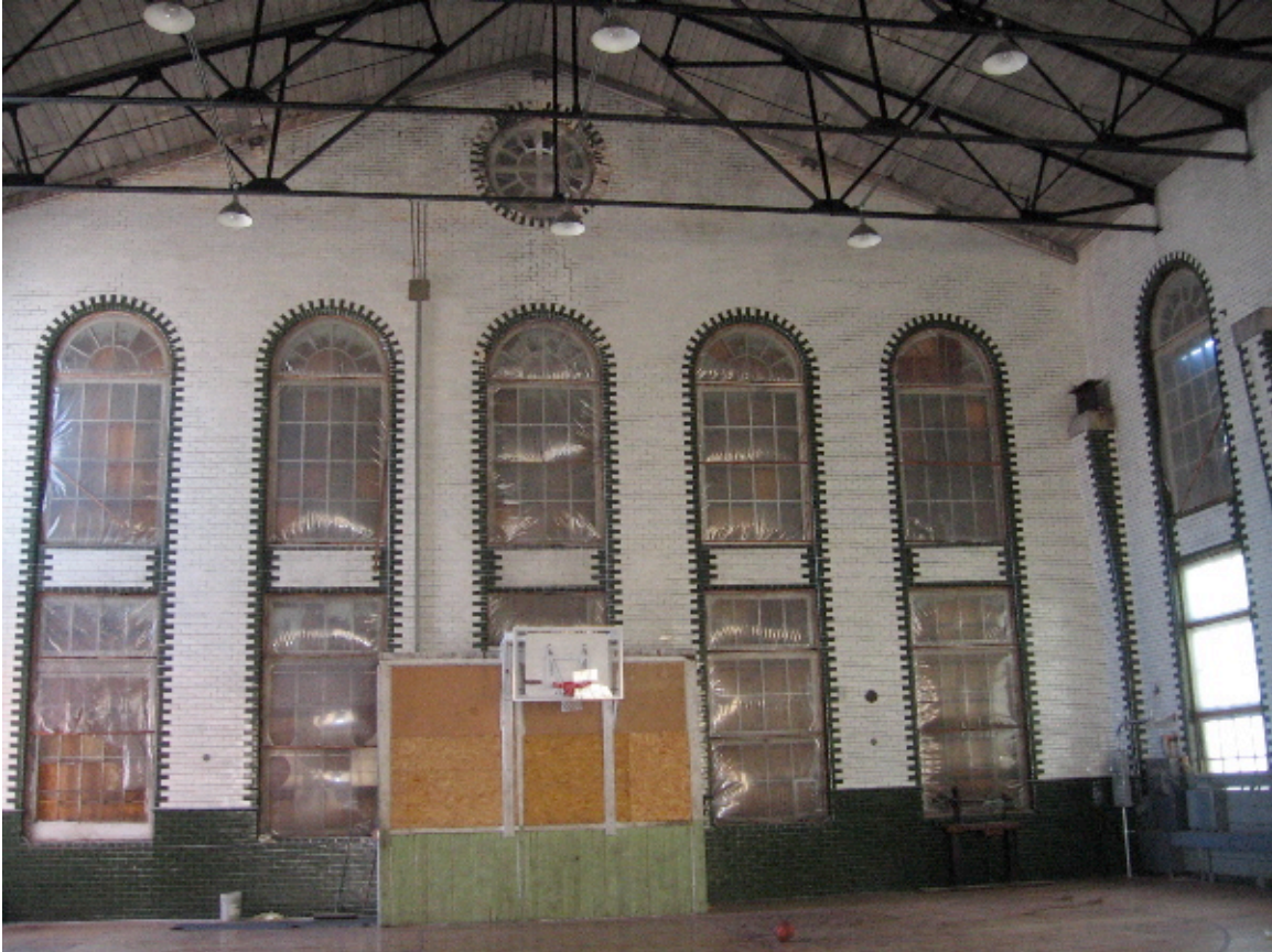
Beneficial reuse of the Nashawena Mills generator room
