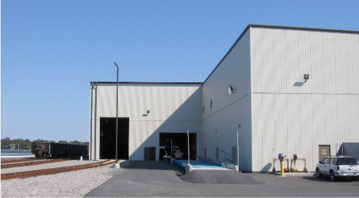
Dewatering facility, with empty train cars on left
