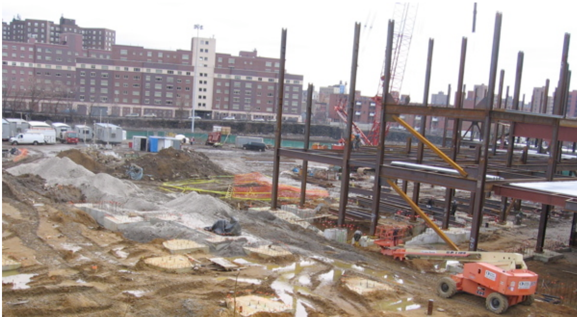
Figure 4: Site Construction (View from Northwest)
