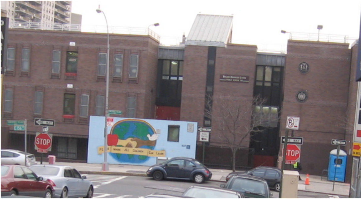
Figure 5: Entrance to Existing School
