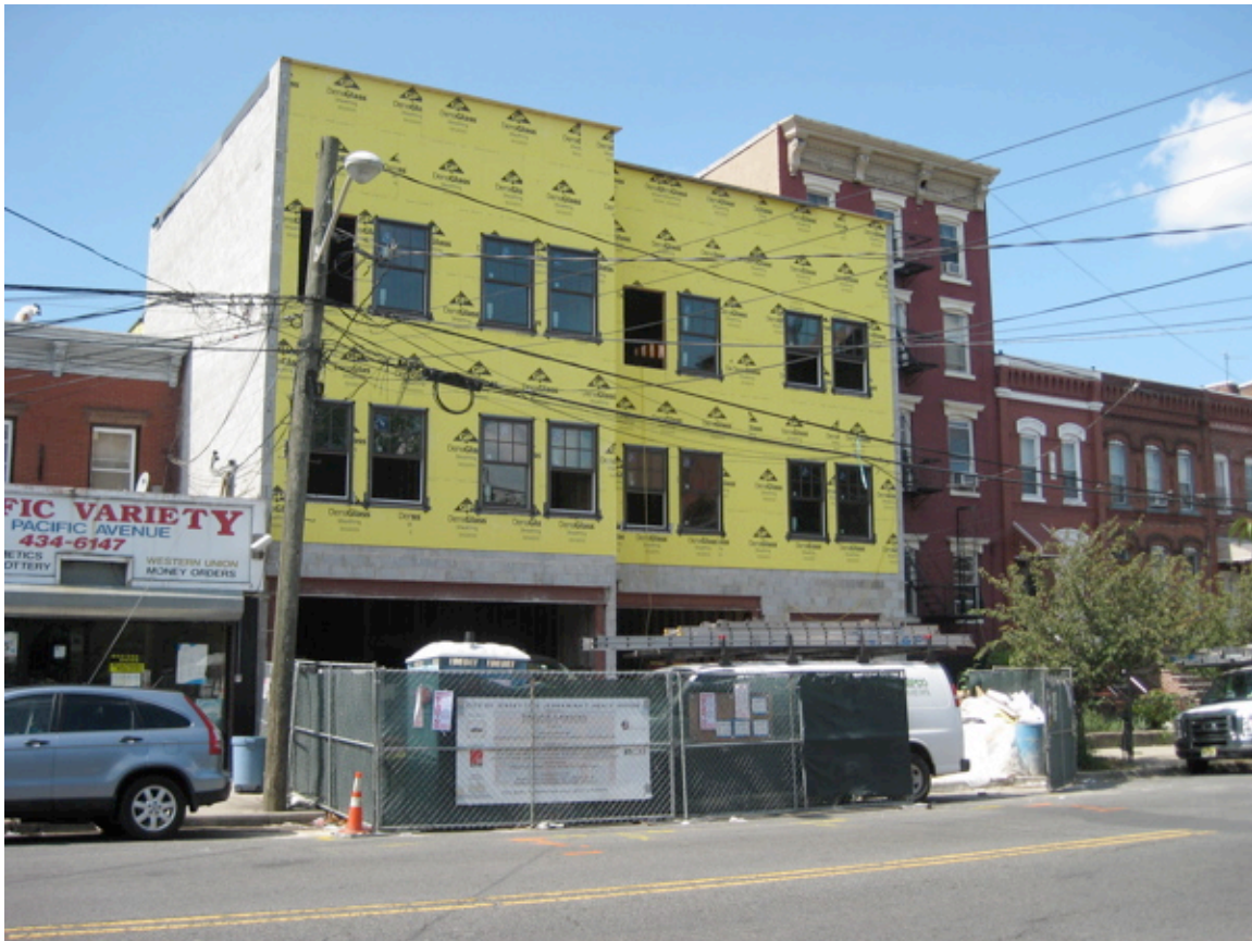
Pacific Landing construction site, August 2012
