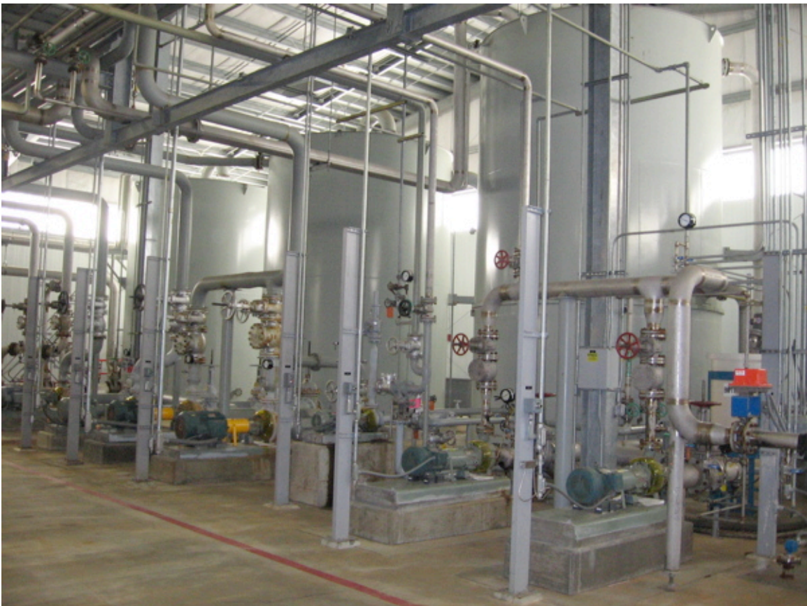
Pump and Treat System at Otis Air National Guard Base, Massachusetts
