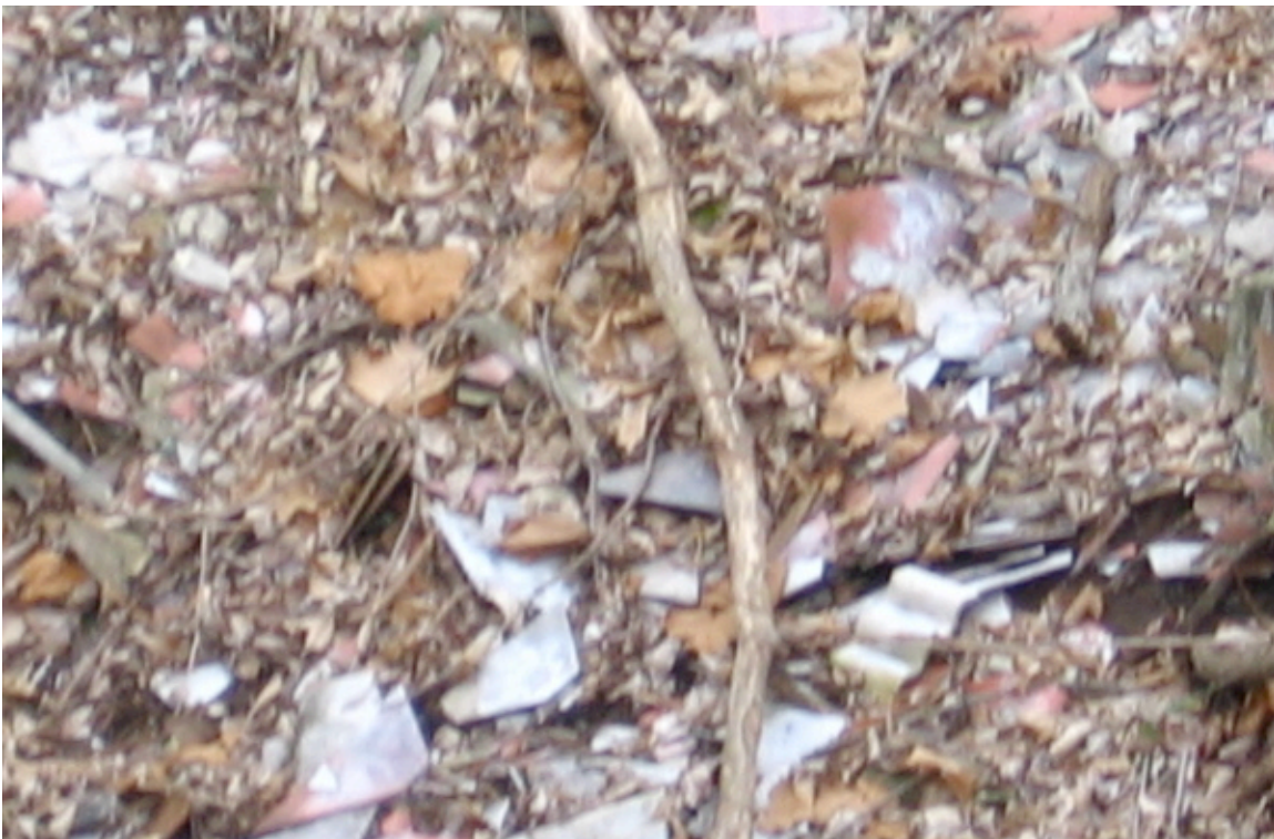
Exposed asbestos waste
