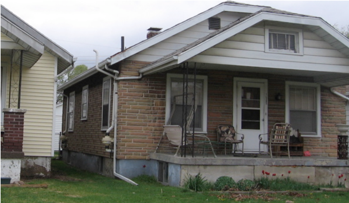
House with Two Subslab Depressurization Systems
